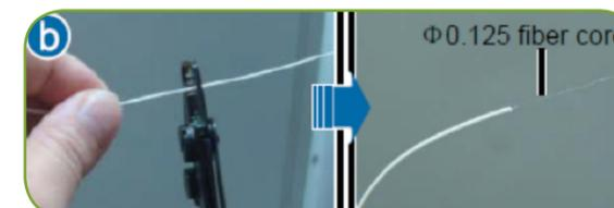
b) Strip the pigtails into 0.125 fibre cores
